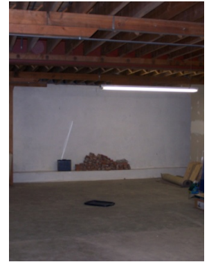
Floor and ceiling
