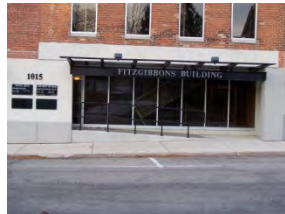
East project entrance
