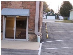
West unit entrance
