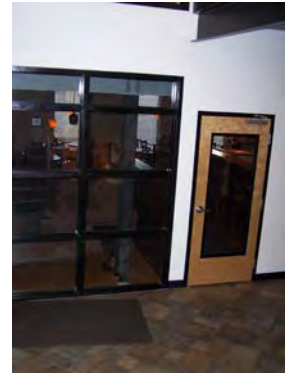
Unit entrance from lobby
