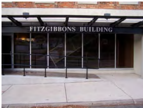
East entrance to lobby
