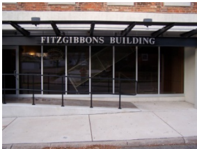
East entrance to lobby
